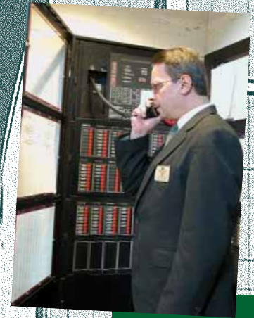
Bank One Center Security Officer JOHN BENLINE announces an emergency evacuation drill from the central console in the main lobby.
